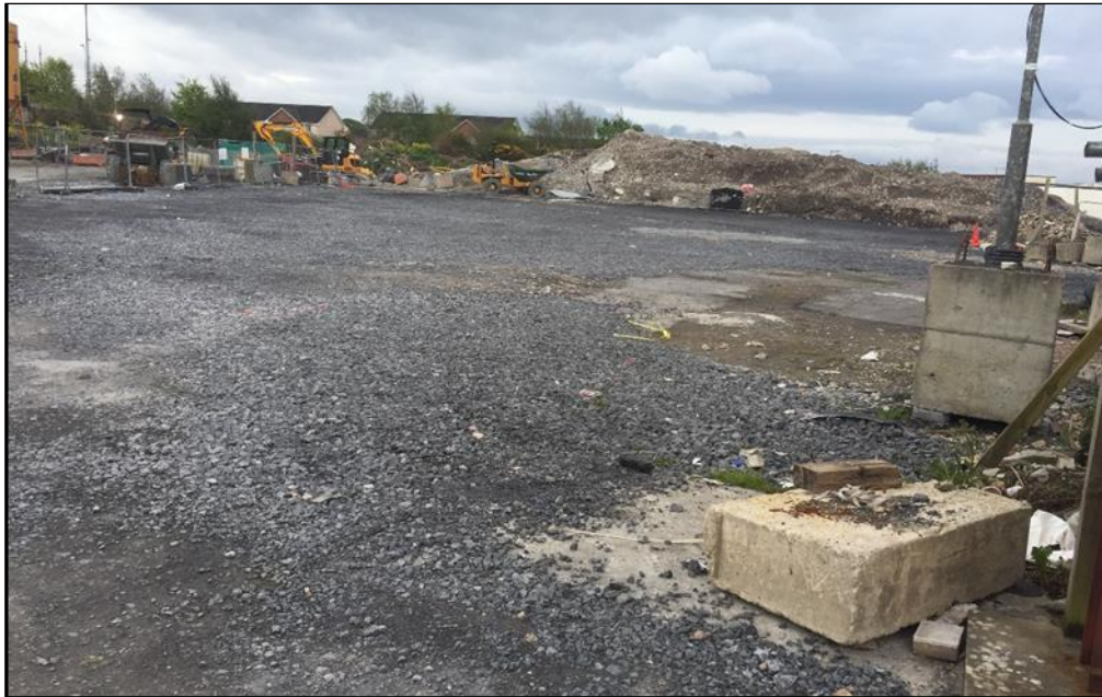
Plate 2.2: Spoil and Bare Ground (ED2)
